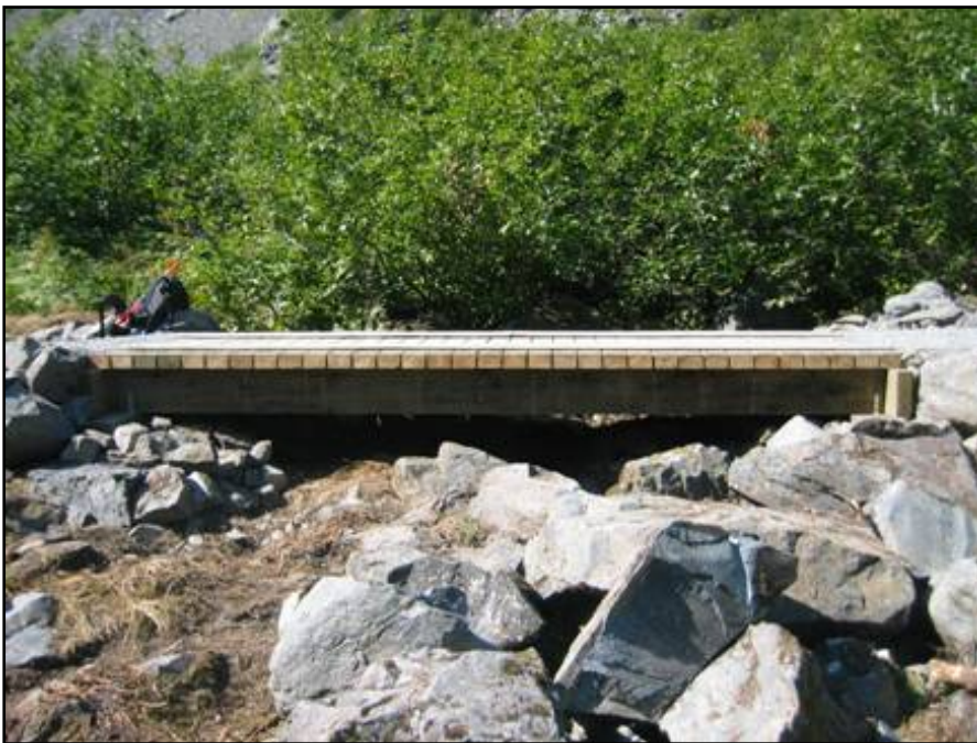
Structure has all the basic structural elements.
