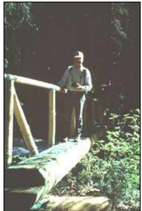
Single span trail bridge over actively flowing water.
