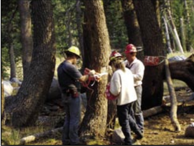
Figure D-19—Strapping explosives to trees.
