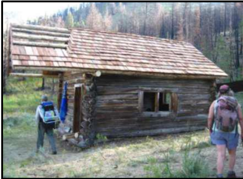
Figure 12. Warm Springs Ranger Station Showing Restoration Work Remaining to be Done.
