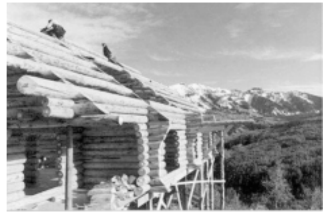
Figure 2—Workers construct an inholder's cabin, which is visible for several miles throughout the West Elk Wilderness, Colorado. Photo courtesy of The Wilderness Land Trust.
