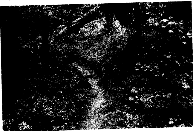
Figure 9.—Trail incision commonly occurs even on moderate slopes if water bars have not been used.
