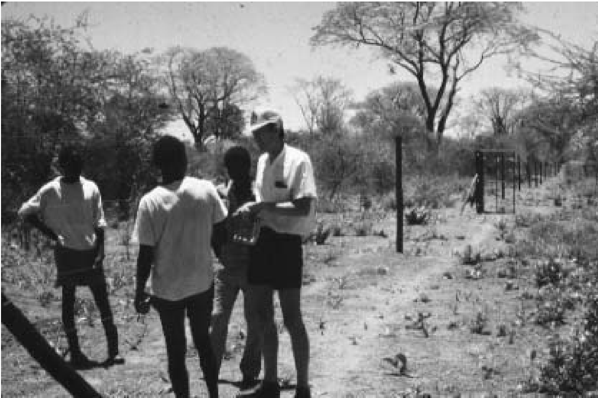
Figure 4 —Developing skills in electrified game fence maintenance, necessary when zoning for wildlife use.
