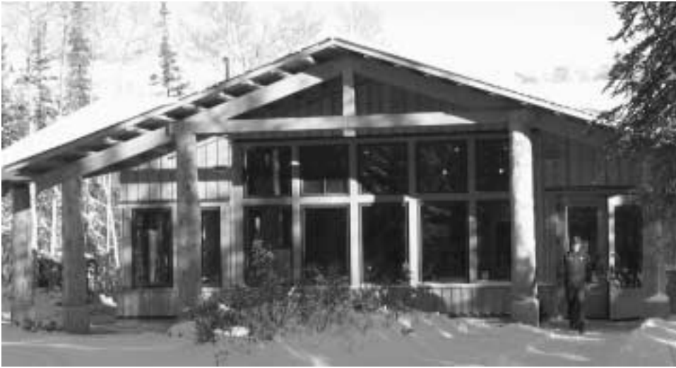
Figure 2—Murie Science and Learning Center, Denali National Park and Preserve, Alaska. Photo courtesy of Fred Bayler and the National Park Service.
